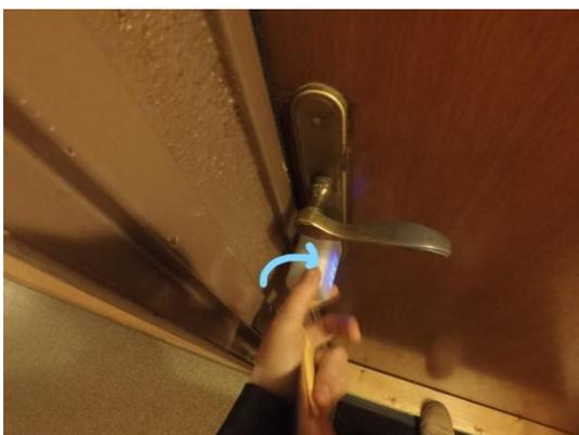
Enter the Smartlock password and push the unlock button, turn the lock to the right, you can now open the door
