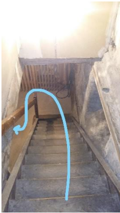
Go down to the cellar with the chain
