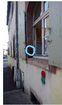
The lockbox is located near the window (Rue des écoles)
