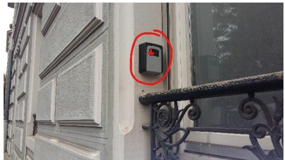
The lockbox is located near the window
